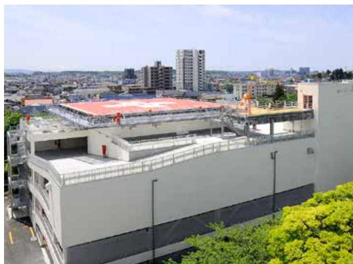
Helipad and Multistory parking lot
