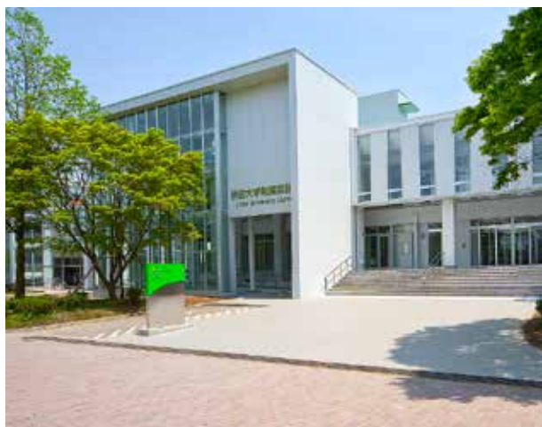
Central Library (main entrance)
