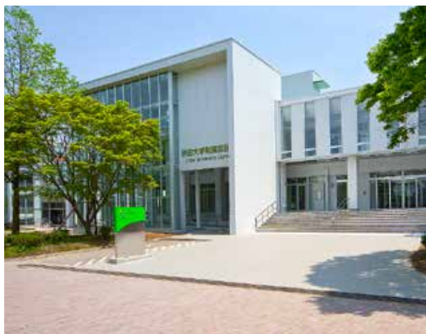
Central Library (main entrance)
