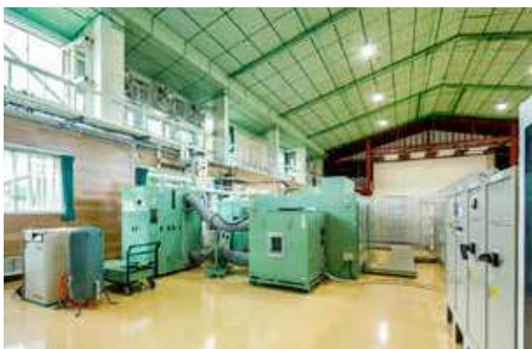
One of the largest motor characteristics testing facilities in Japan *Establishment of Evaluation Laboratory for Next Generation Motors
